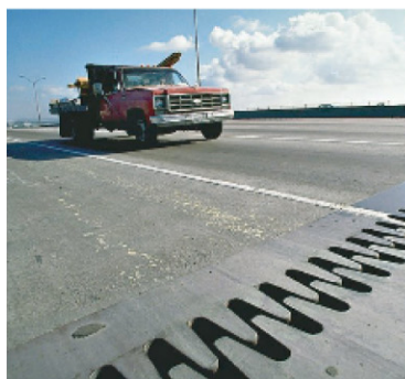
FIGURE 13-3 Expansion joint on a bridge.
