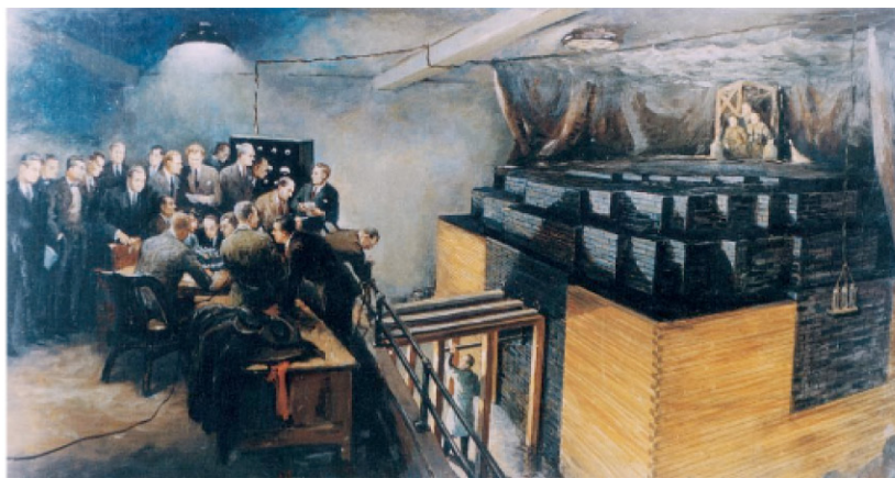
FIGURE 31-5 Color painting of the first nuclear reactor, built by Fermi under the grandstand of Stagg Field at the University of Chicago. (There are no photographs of the original reactor because of military secrecy.) Natural uranium was used with graphite as moderator. On December 2, 1942, Fermi slowly withdrew the cadmium control rods and the reactor went critical. This first self-sustaining chain reaction was announced to Washington, by telephone, by Arthur Compton who witnessed the event and reported: “The Italian navigator has just landed in the new world.” Gary Sheahan, “Birth of the Atomic Age,” Chicago (Illinois); 1957. Chicago Historical Society, ICHi-33305.
