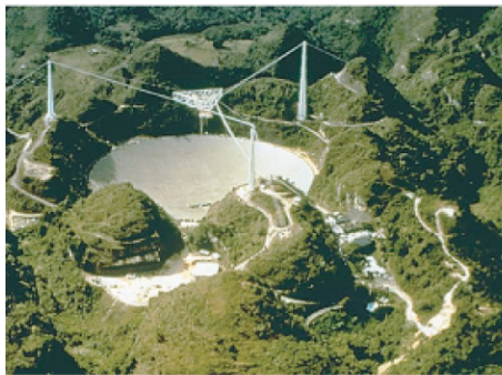
FIGURE 25-32 The 300-meter radiotelescope in Arecibo, Puerto Rico, uses radio waves (Fig. 22-8) instead of visible light.
