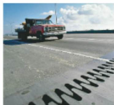
FIGURE 13-3 Expansion joint on a bridge.
